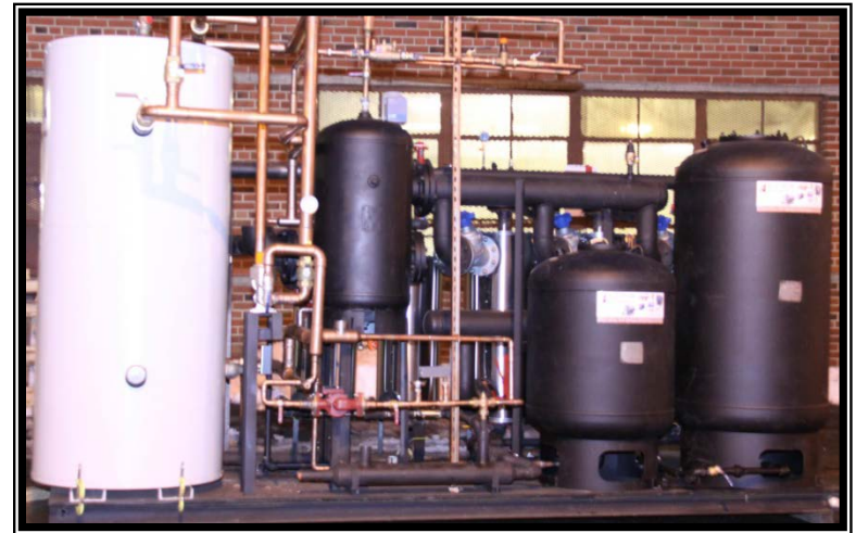
Triplex Skid Package: Heating-Hot Water-Pumping-Expansion-Air Separation
